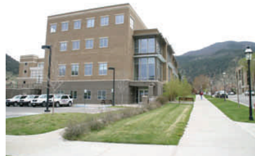
City Hall Police Dept Entrance (West End of Building)
